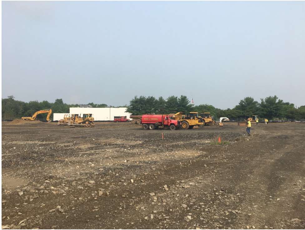
Construction workers begin working on the project following the groundbreaking.
